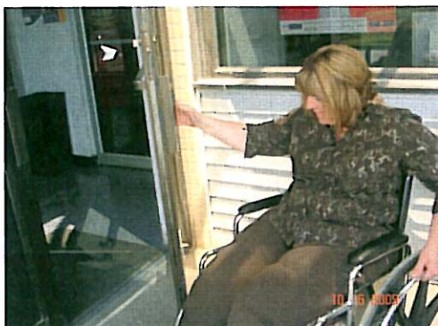
Councillor Olson struggles to open the heavy doors at the Post Office. A simple solution would be to install hold open automatic doors.
