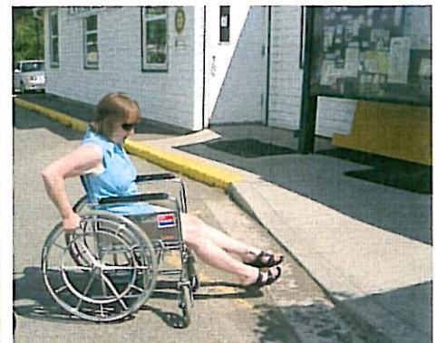
Councillor Benedict gets a run at it while trying to access the Chamber of Commerce building. The lip on this ramp is too high to easily get over with a manual wheelchair.
