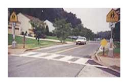
A push button at either end of the crosswalk activates six high intensity yellow lights that flash once per second for 30 seconds. The staggered placement of TS230 fixtures maximizes visibility.
