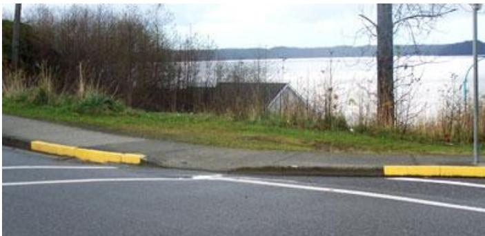
There are a number of sidewalk curb cuts throughout town that try to service two crosswalks with a single cut, such as this one pictured left. This forces wheelchairs to enter vehicle traffic to align with the cutout. When and where possible, the city should augment these cutouts to accommodate both crosswalks in a head-on orientation.
