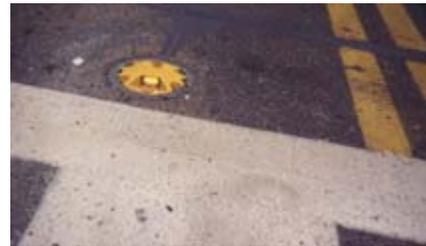
*The TS230 is only 8" in diameter and will withstand a dynamic load of eleven tons. The fixture slopes from 0 - .39" above the roadway, so that bicycles and snow plow blades ride over it without hindrance. The caution-yellow light flashes in both directions.*
